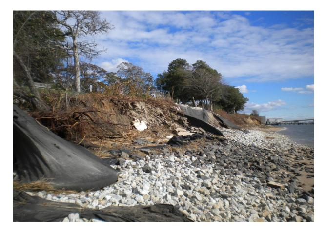
The City of Somers Point has an excellent example of a living shoreline at John F. Kennedy Park which overlooks that Green Egg Harbor River on Broadway. This park was prone to erosion and sustained significant damages as a result of Superstorm Sandy. The City Engineer designed a rock filled gabion system to repair and prevent future erosion events. Funding was secured from FEMA for this project.
